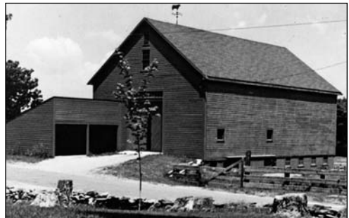
The Barn at Whittier's Birthplace is in need of extensive repairs.
